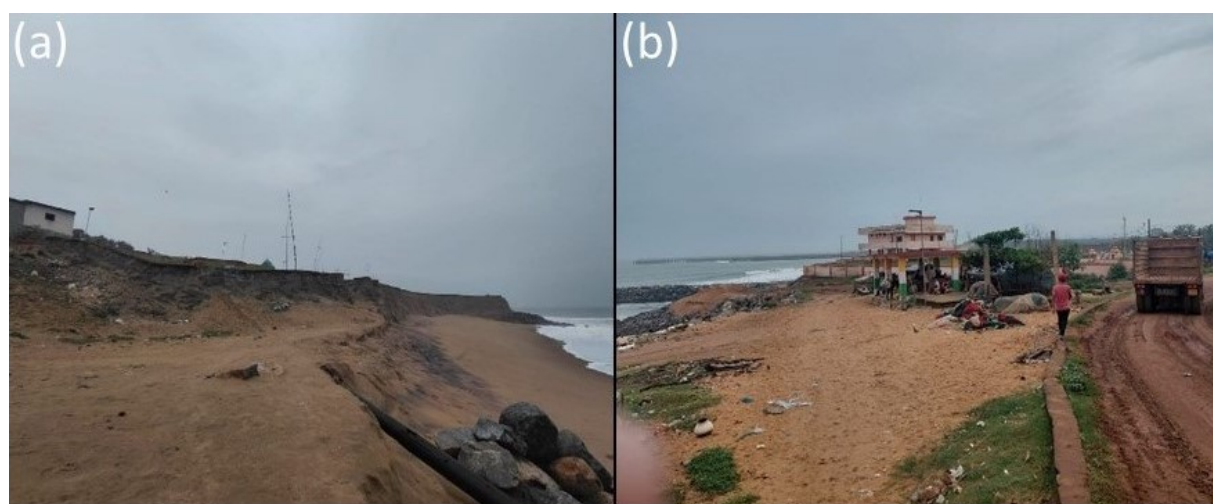
Fig. 7. A coastal road was washed away at the sea coast near Arjyapalli census town. (b) The marine police station standing on the verge of the sea coast at Arjyapalli census town, indicating the future threat to the settlements.
